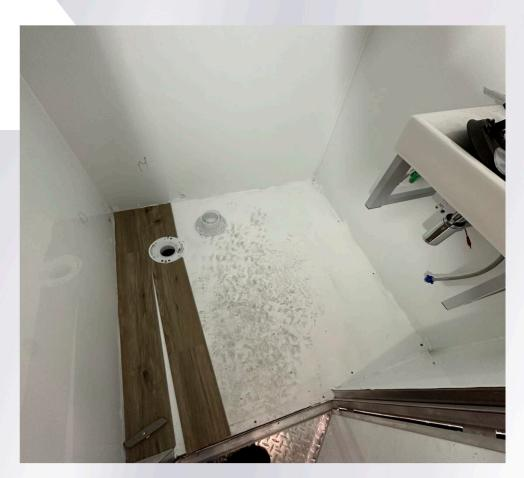
The trailer floor is built of a heavy duty metal chassis, apart we installed a fully waterproofed floor to protect it from water.
